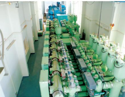
The first shipment of the gas insulated switchgear for the 220 kV facility arrived on 6 March 2012. The installation works and testing on-site lasted until 30 August 2012. The gas insulated switchgear in SS Plat is the first of a kind in the Republic of Croatia.
