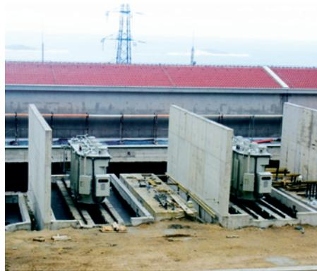
Two 220/110 kV, 150 MVA transformers were delivered to SS Plat on 20 June 2012. Installation works and on-site testing was completed by 8 December 2012.
