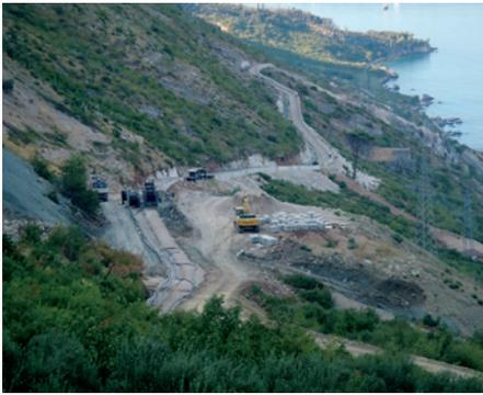
Construction works on connecting cable lines began on 24 March 2011, while the installation works began on 31 July 2012. The total of 7.850 m of 220 and 110 kV cables, and 39.024 m of 35 and 20(10) kV cables were buried in SS Plat and the connecting cable routes.
