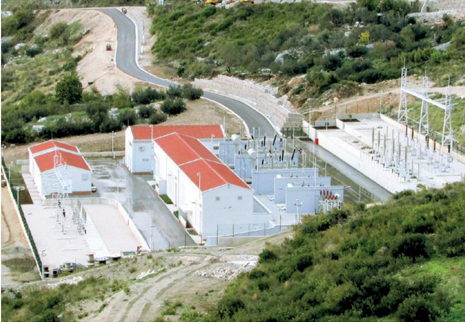
the 220/110/35/20(10) kV switchgear is situated, comprising two 220/110 kV autotransformers, 150 MVA (AT1 and AT2), a 110/35 kV, 20 MVA (TR1) and a 110/20 kV, 20 MVA (TR2) transformer, and an 35/20(10) kV, 16 MVA interconnecting transformer. Unit auxiliary transformers 35/0.4 kV, 630 kVA and 20(10)/0.4 kV, 630 kVA are situated on the ground floor of the management and control facility.
