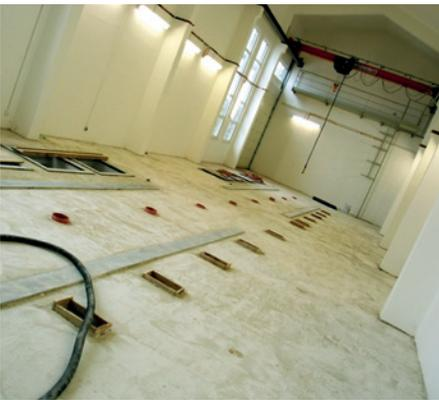
The erection of electric power facilities in SS Plat began on 15 February 2011 when the grounding grid was installed during construction works. The work on electrical installations and lighting began on 10 January 2012 in the room wherein the gas insulated switchgear was to be placed in the 220 and 110 kV facility. An overhead travelling crane with load capacity of 5t was installed in the room.
