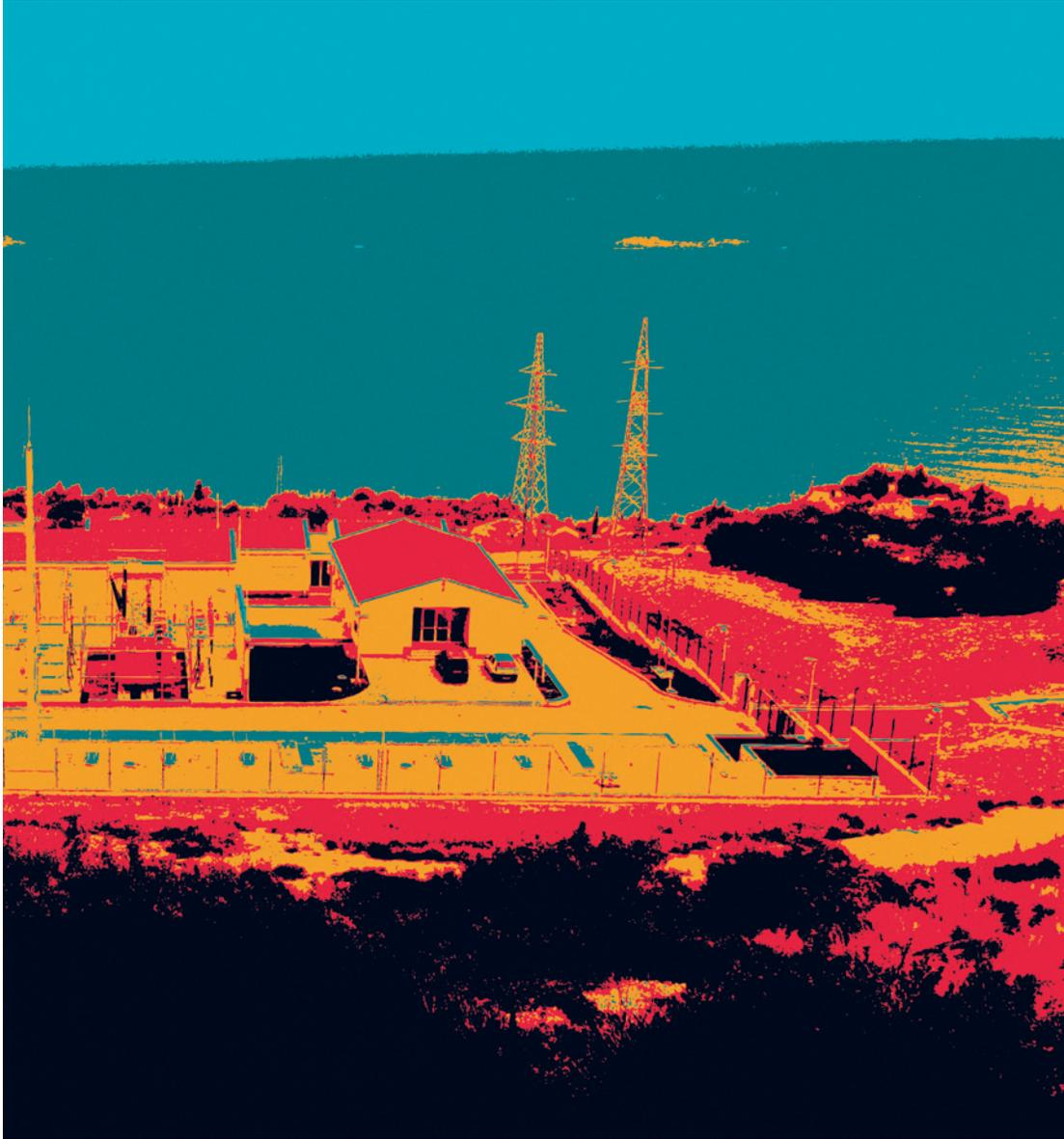
The construction of the 220/110/35/20(10) kV Plat substation and the connecting lines began on 22 October 2010. The construction was characterised by demanding field work in the area potentially prone to landslides. The first concrete was placed in the substation on 14 January 2011. The total of 57.000 m<sup>3</sup> was excavated for foundations, and the total of 6.839 m<sup>3</sup> of concrete was used.
